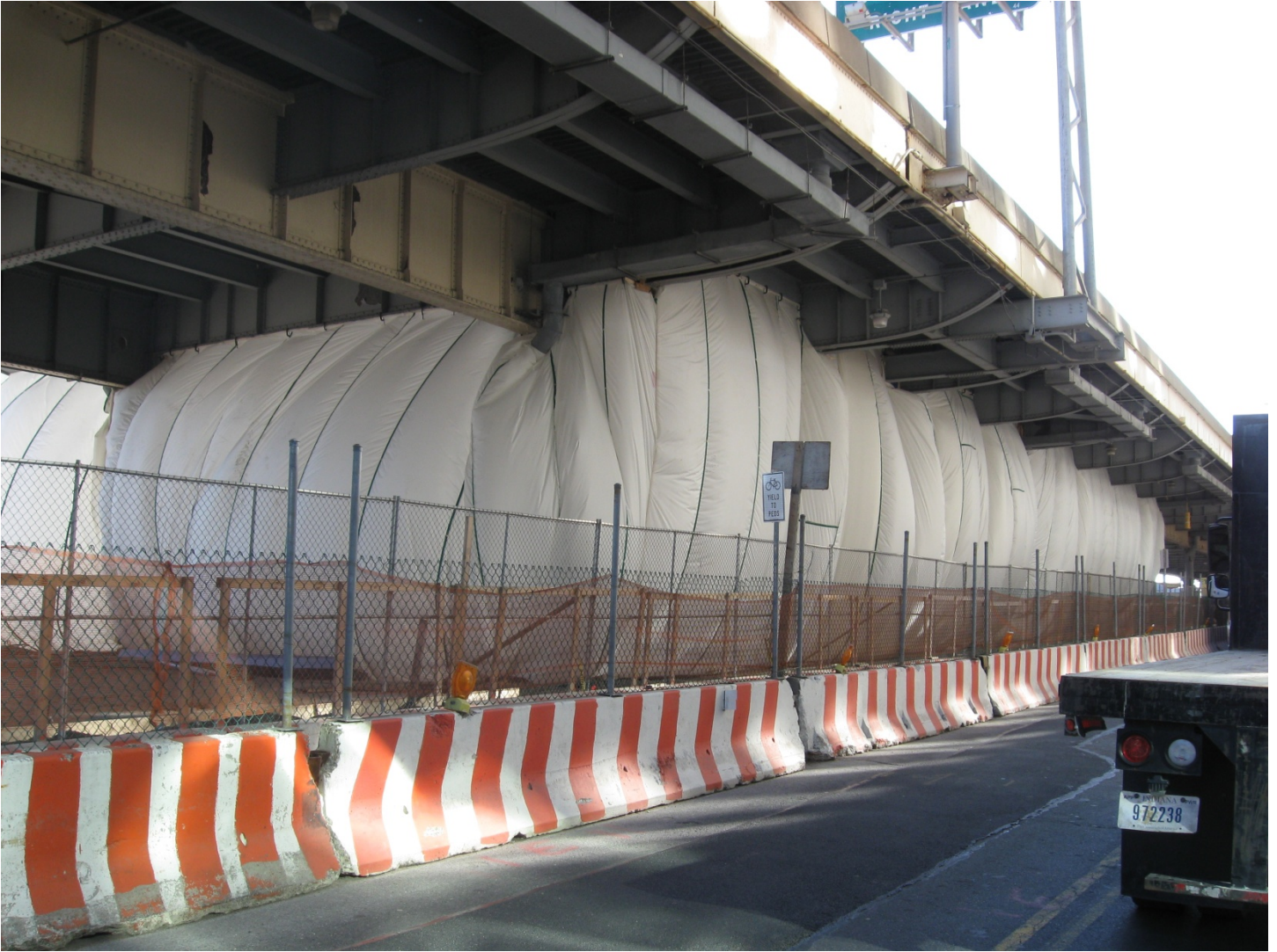
Containment Tarpaulins To Grade
