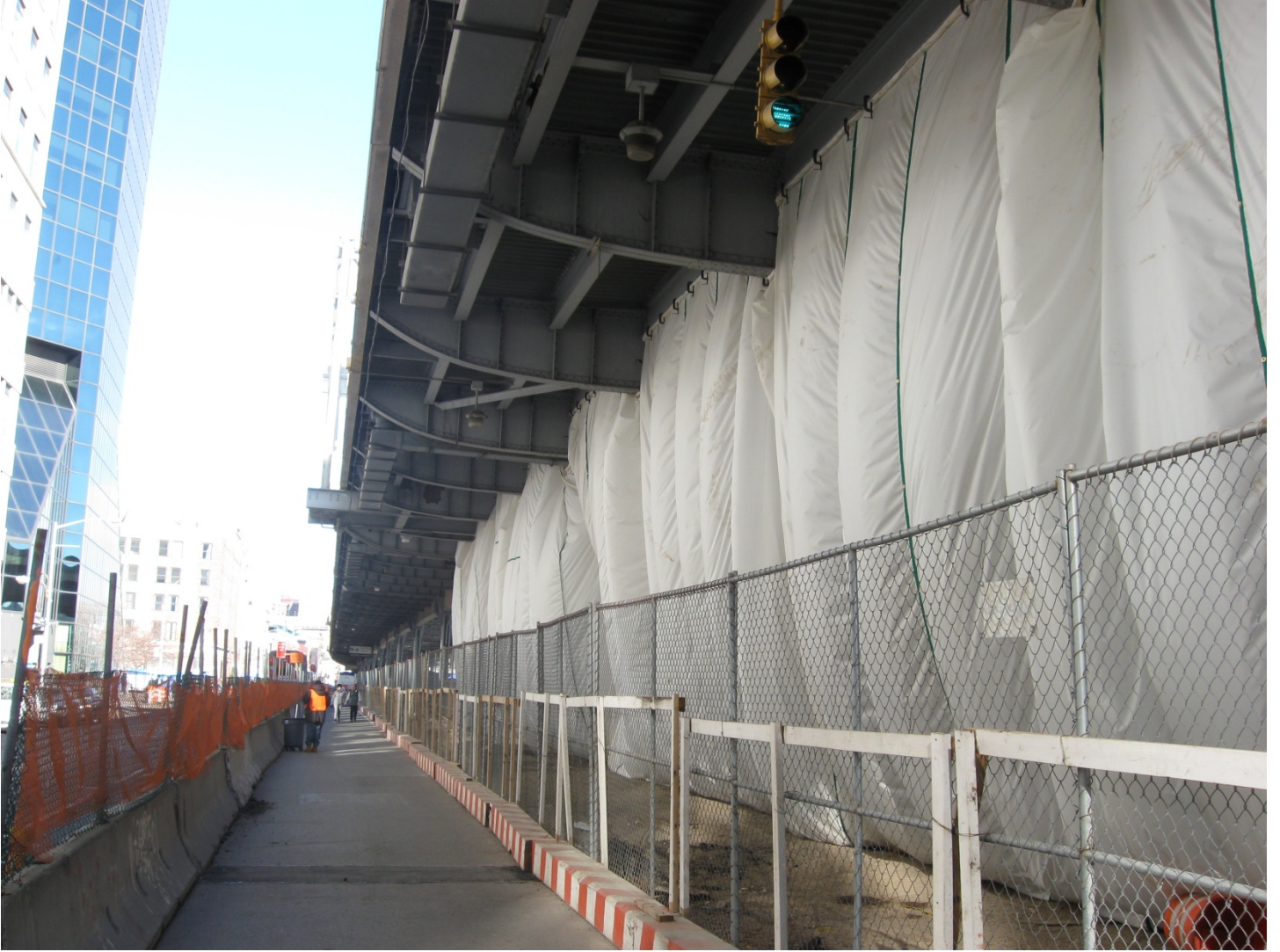
Containment Tarpaulins To Grade
