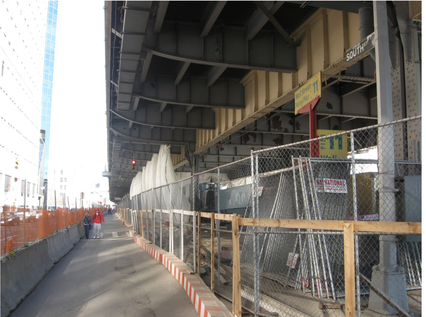
Containment Tarpaulins To Grade
