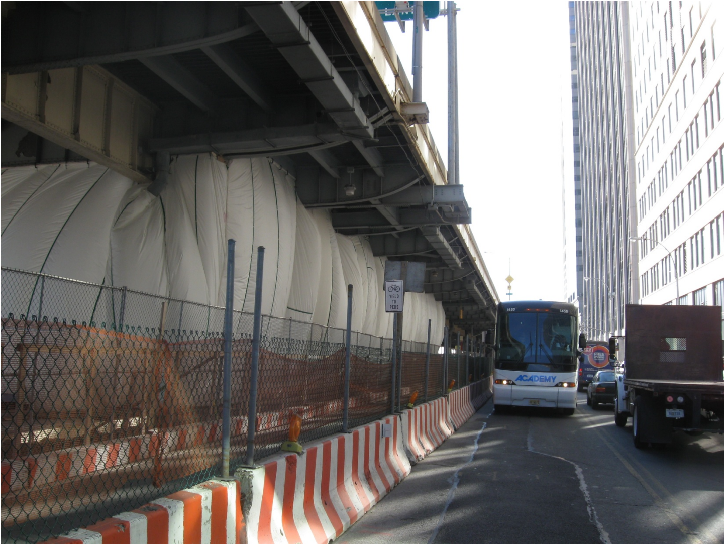
Containment Tarpaulins To Grade
