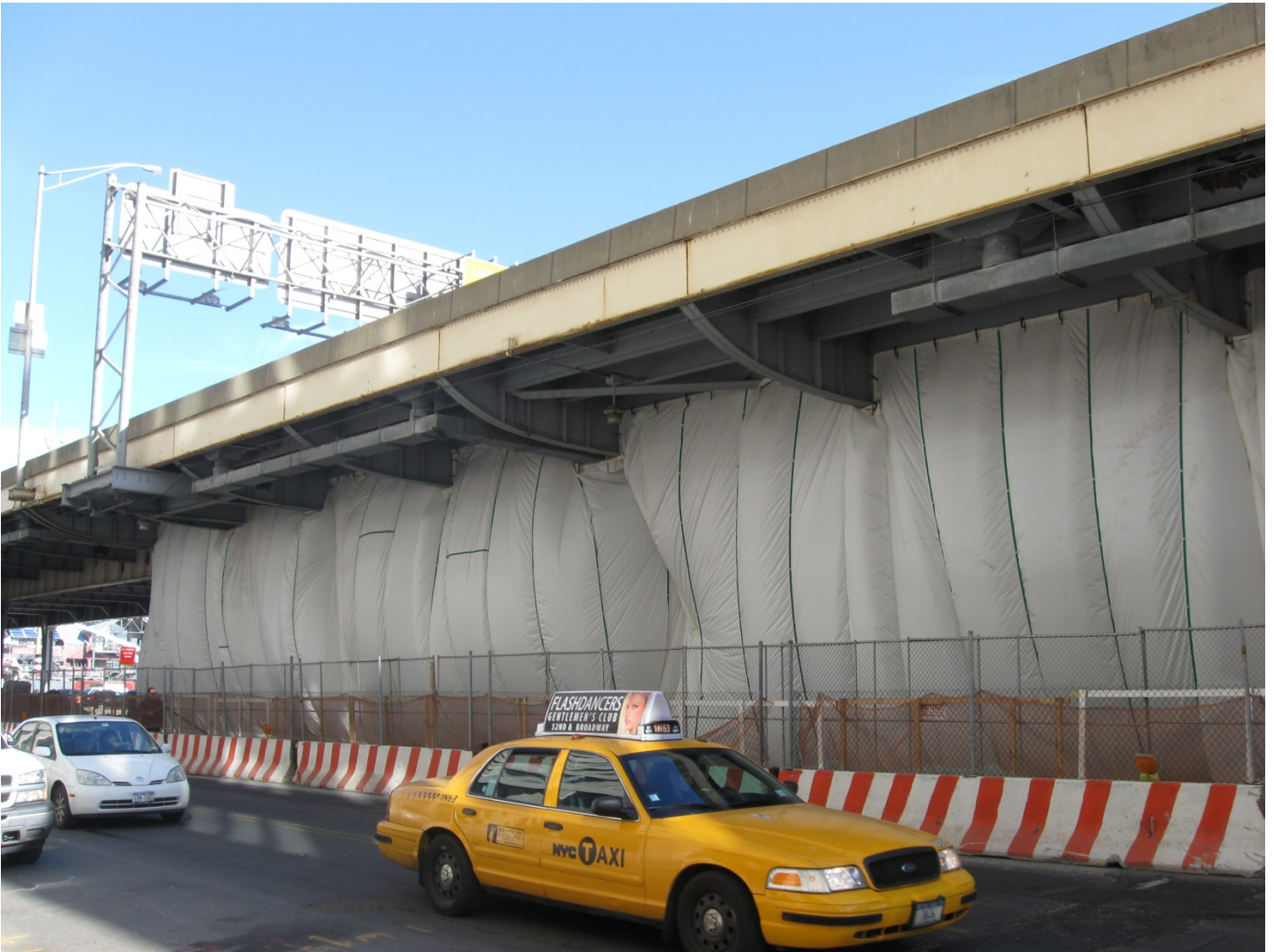
Containment Tarpaulins To Grade
